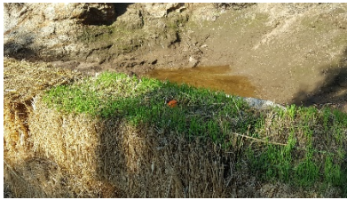
Along the road, gabions replace higher-upkeep straw bales - shown below. These mitigate runoff into neighbors' yards and homes.
