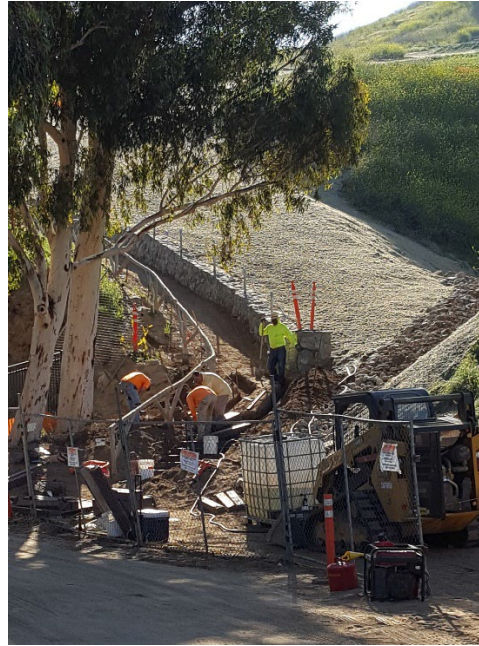
Along the road, gabions replace higher-upkeep straw bales - shown below. These mitigate runoff into neighbors' yards and homes.
