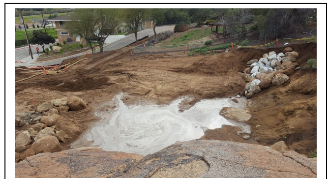
Photos at right are of “in progress” City Public Works and Parks Departments’ catch-basin project to control runoff from Glenwood / San Andreas corner of Mt. Rubidoux Park.
